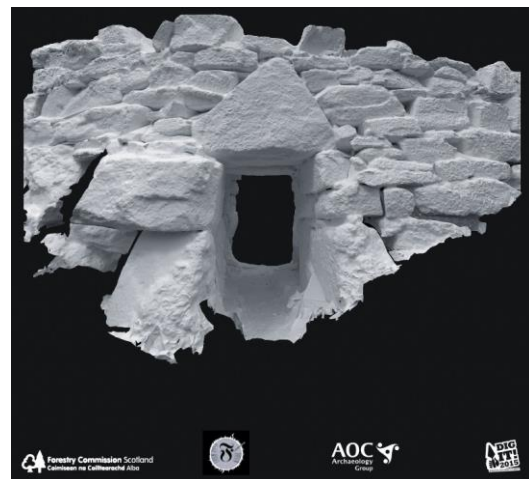
Caisteal Grugaig Broch, Glenshiel. To enhance the existing records of the site, Forest Enterprise commissioned a new measured survey using modern techniques, including laser scanning technology. This detail shows the huge triangular lintel over the low entrance passage. © Forestry Commission
